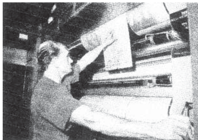
Figure 8. Mounting an offset plate on a planographic press.
